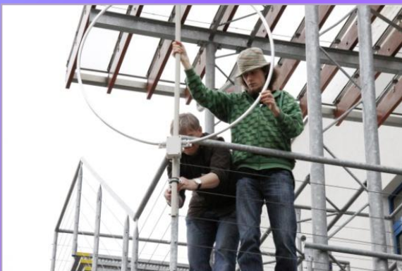
Instalation of SID monitor antenna – detector of radio VLF disturbances as alternative method to detect gamma-ray bursts
